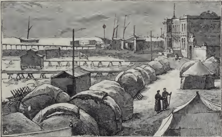
GOVERNOR'S HOUSE AND STORES AT KRASNOVODSK.
